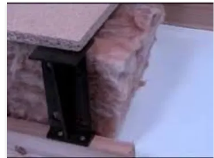
Loft Boarding on Leg Floating Floor £58.00 per square metre
